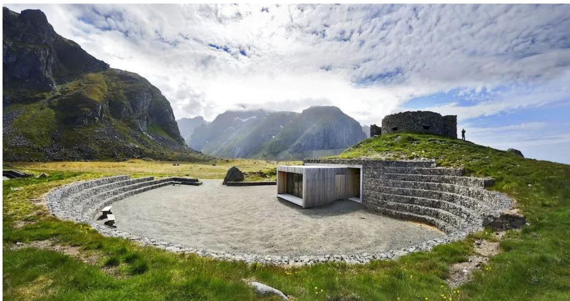
Rest Area in Eggum, Norway, by architect Snøhetta along the Scenic Route Lofoten along EuroVelo 1 © Jarle Waehler - Statens vegvesen
